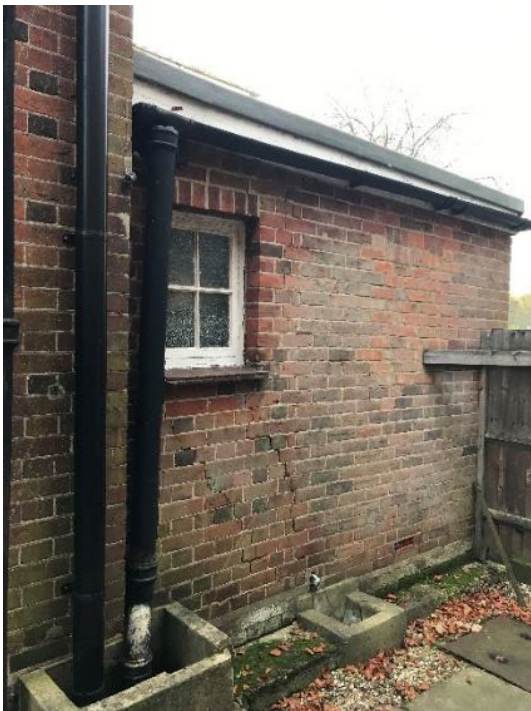
Fig. 37: The single-storey section of the south-east pavilion, showing the area of original brickwork (in the area of the window) which once supported a balcony above. This block was altered and extended in the 1930s. (© Emily Cole)
