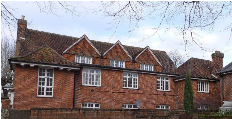
Fig. 31: The Hall from the south, showing well-preserved features including clay tiles, dormer windows with tile-hung gablets above, eaves brackets, windows and chimneys. (© Emily Cole)
